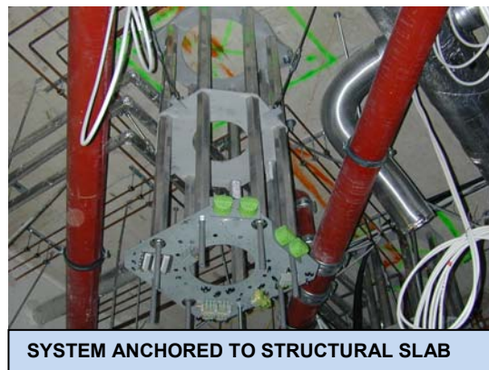
Picture #2) TRUMPF EMS Mounting System – Attachment Methods
