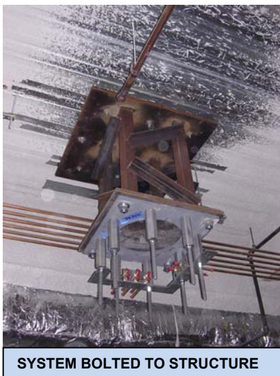
Picture #2) TRUMPF EMS Mounting System – Attachment Methods
