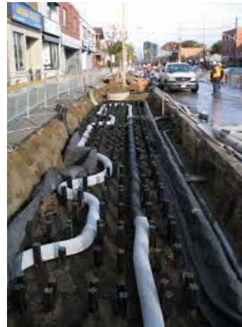
Figure 6-6 - Stormwater tree trench with soil cells
