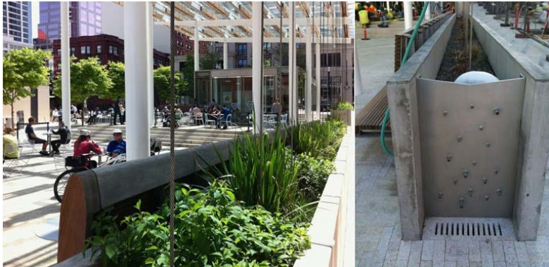
Figure 6-1 - Bioretention Planter - Portland Director Park (stormwater planter watered by canopy runoff. Rain chains into planter with overflow spouts)
