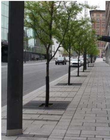
Figure 6-5 - Stormwater tree trench with paving
