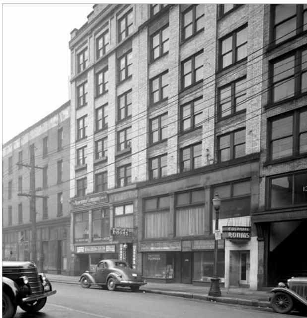
The Gastown Hotel built in 1912-1913, Sharp & Thompson Architects.
