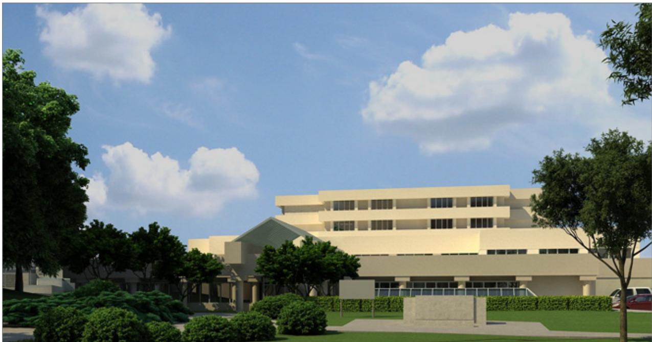
Front entrance to the future renovated lobby of the Surrey Pretrial Services Centre.
