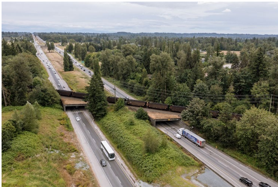
Figure 1 – EXISTING HIGHWAY 1 UNDERPASS
