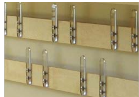
FIGURE 12 - NOTE: THIS EXAMPLE SHOWS ACRYLIC HOOKS. STAINLESS STEEL IS REQUIRED.
