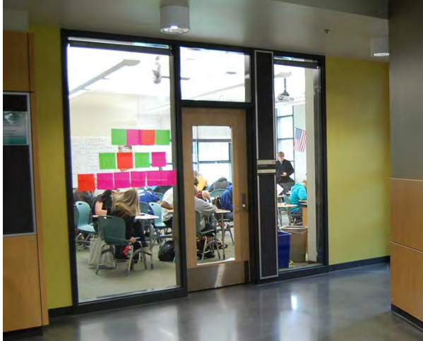
Picture 15 – Example of Visibility into Classrooms by Entryway, Note Rolling Blinds for Option of Privacy, Meadowdale Middle School
