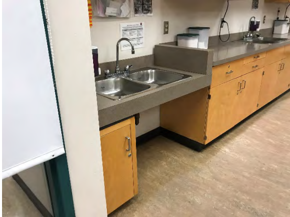
Picture 1 – Example of Accessibility in a Home Economics Classroom, Magee Secondary School
