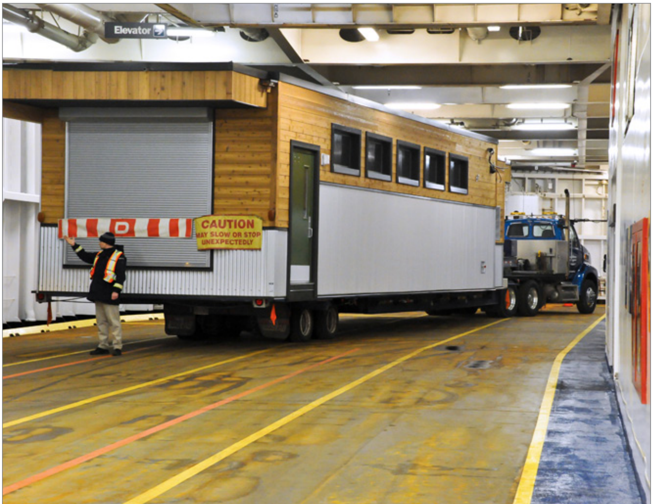
One section of a modular classroom unit, destined for a school site in Sooke, is loaded onto a BC Ferry.
