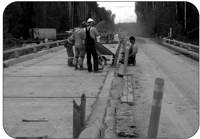
Construction on the Snake River Bridge joint
