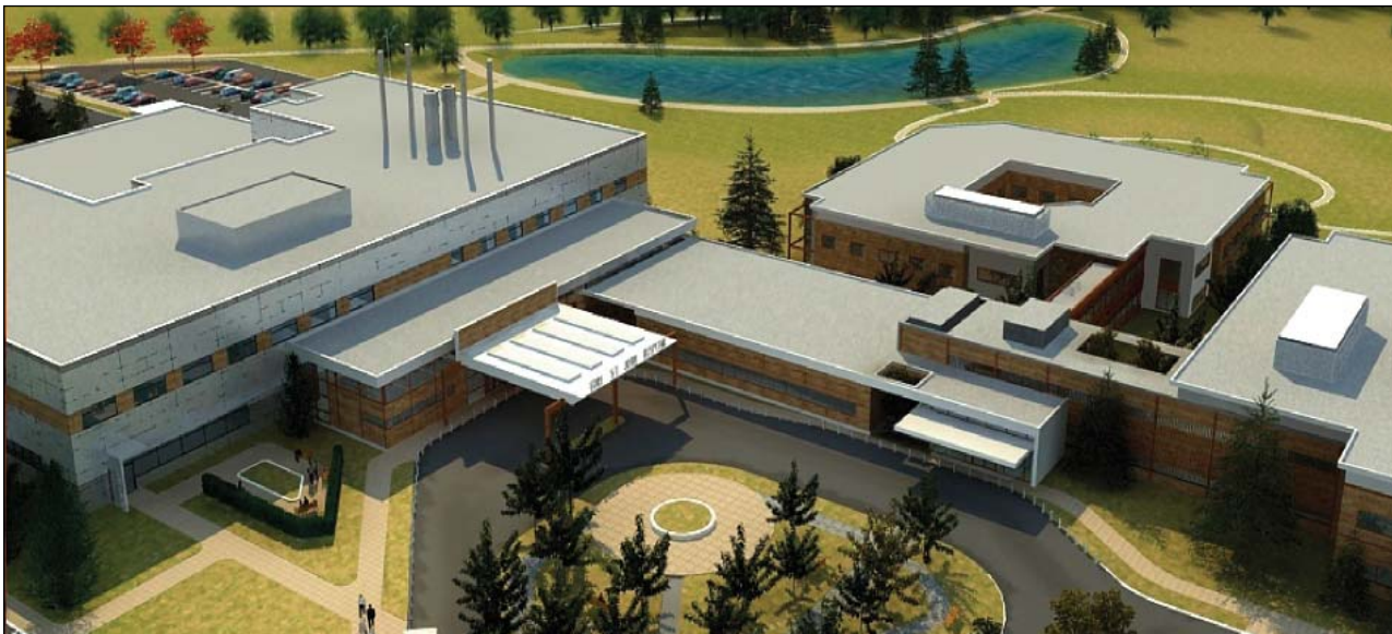
Aerial view of the entrance to the hospital and residential care facility. In the background, a retention pond for excess storm water and snow-melt collected from the roof is part of the storm management program.
