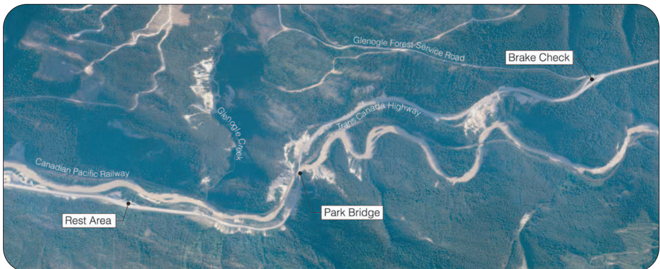
Phase 2 of the Park Bridge and Approaches
